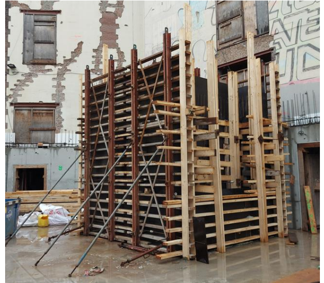
2: Bekisting liftkern
